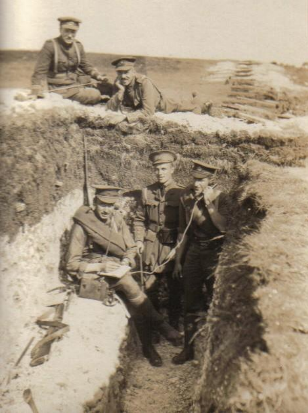
Telephone station, practice trenches, Barham, Kent.
