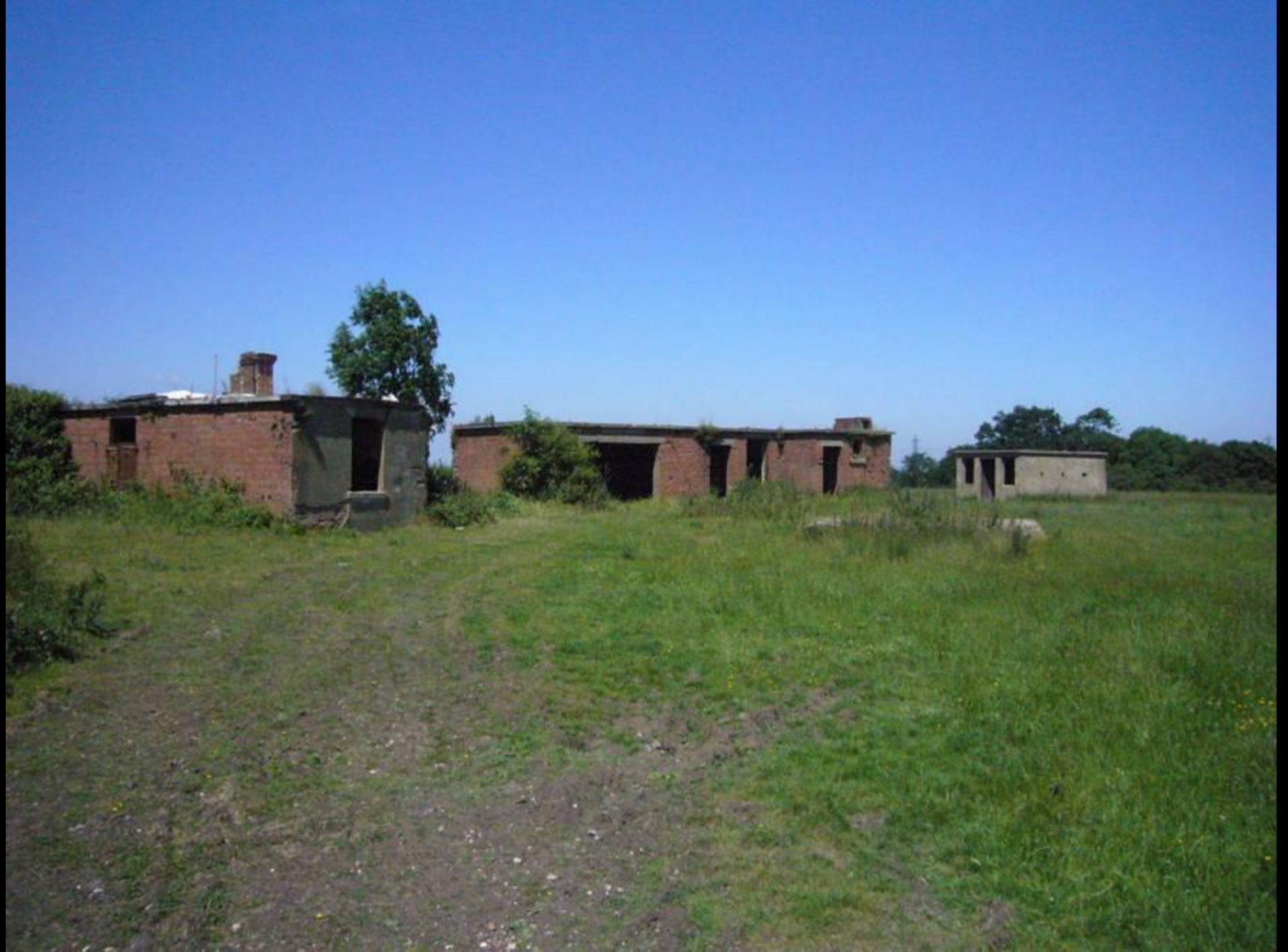
Lodge Hill, Kent, anti-aircraft battery: defensible barracks
